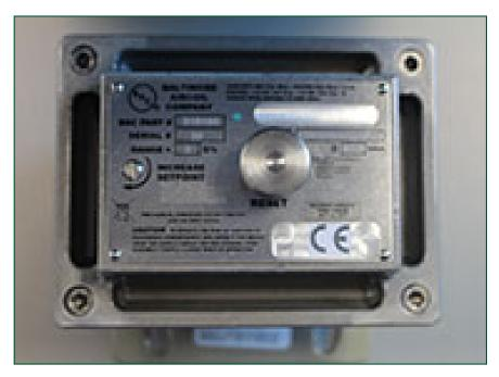
The switch **detects excessive fan drive vibration** caused by fan icing or any mechanical fault. Although factory mounted, the switch point is adjusted on-site during installation and start-up.
