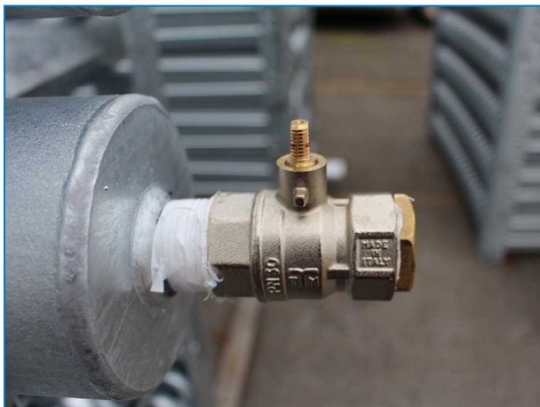
Upper coil connection with pressure release valve on closed circuit cooling towers with connections bigger than ND100.
