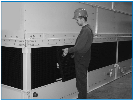
Remove combined inlet shields
